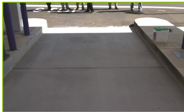
Bank drive-thru AFTER concrete cleaning service
